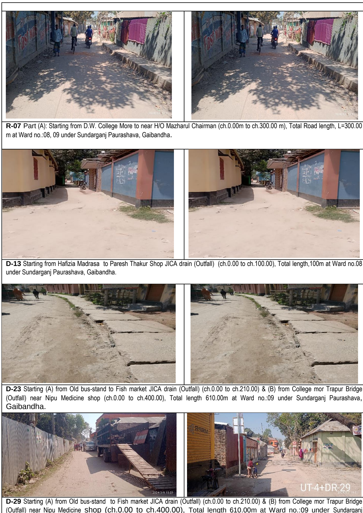
Figure 3:Existing Roads and Drains Picture
